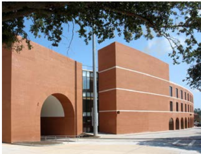
Roberts Stadium - South Stands completed 2008
